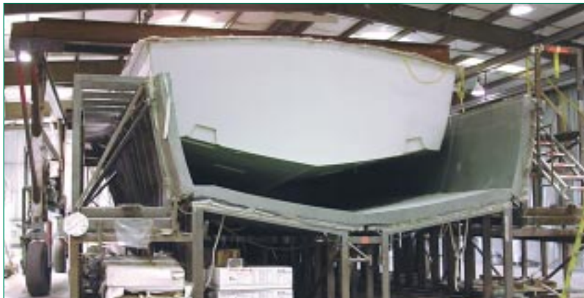
Demolding the hull of the second 81.5 at the Sea Force IX facility.
